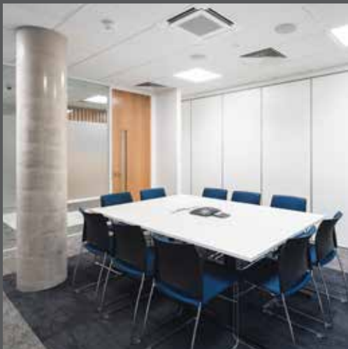
A folding acoustic wall can separate two meeting rooms or be folded to create one large space
