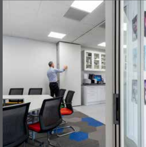
Foldable wall functions as a partition between the laboratory and meeting room or creates an open plan layout.
