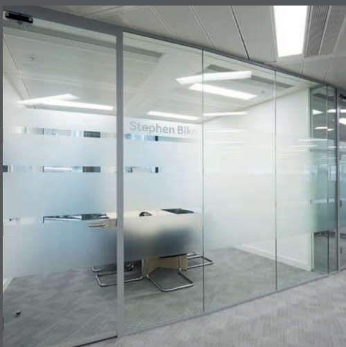
Manifestation was used on the glass partitioning to show who occupied each office
