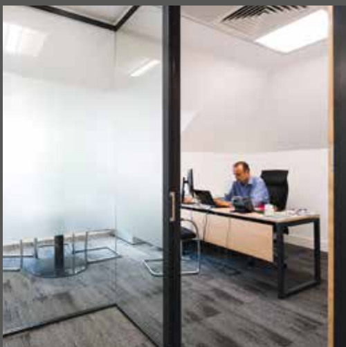
One of the offices - glass partitioning with manifestation and a dark grey frame.
