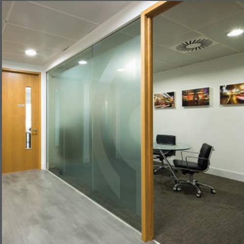
New carpet tiles were laid down in the conference rooms
